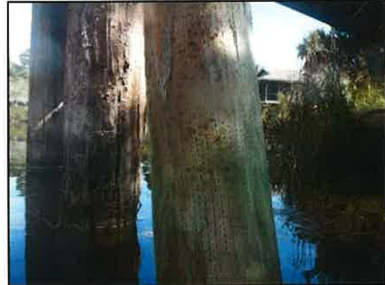
Photo 5-9: View of salt damage on southern battered pile, bent 4
