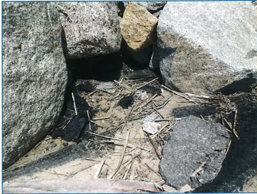
Photograph 3: Station 12+00 – Approximate 3' Diameter Depression Adjacent to Roadway and Evidence of Water Coming Through Revetment
