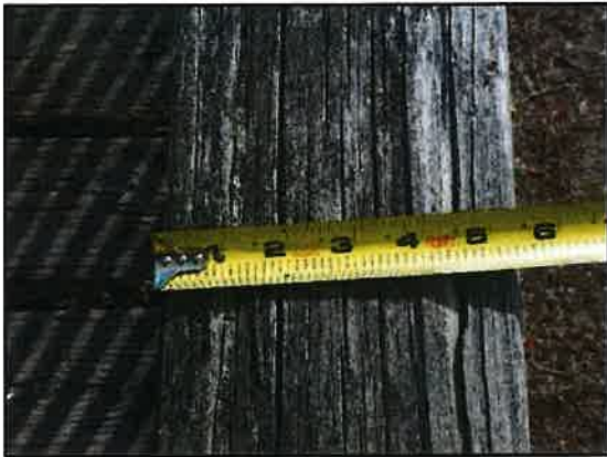
Photo 5-4: View checking on railing
