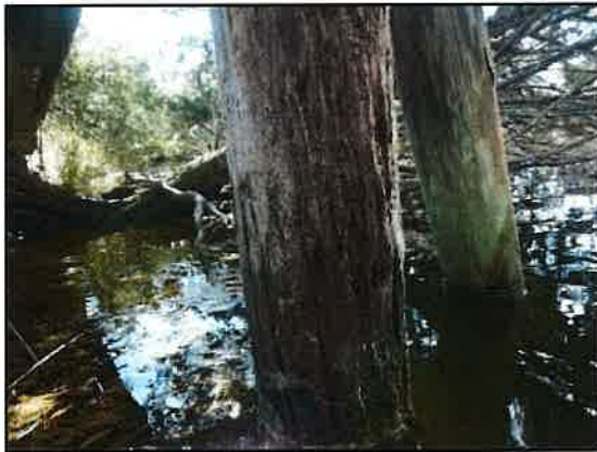
Photo 5-8: Typical view of rot at waterline on pile
