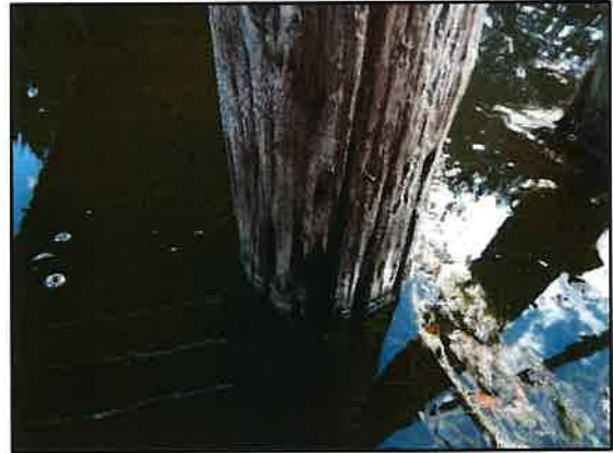
Photo 5-7: Typical view of rot at waterline on pile
