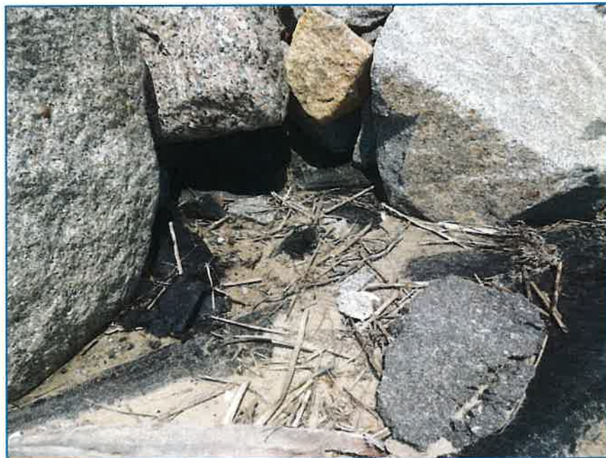
Photograph 2: Station 11+55 – Exposed Filter Fabric and Evidence of Water Coming Through Revetment
