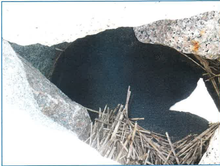
Photograph 1: Station 11+00 – Exposed Filter Fabric in Minor Depression and Evidence of Water Coming Through Revetment
