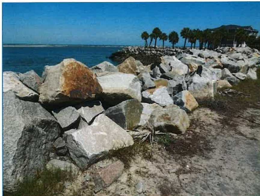
Photograph 4: Station 23+50 to 24+00 - Apparent Settlement of the Revetment
