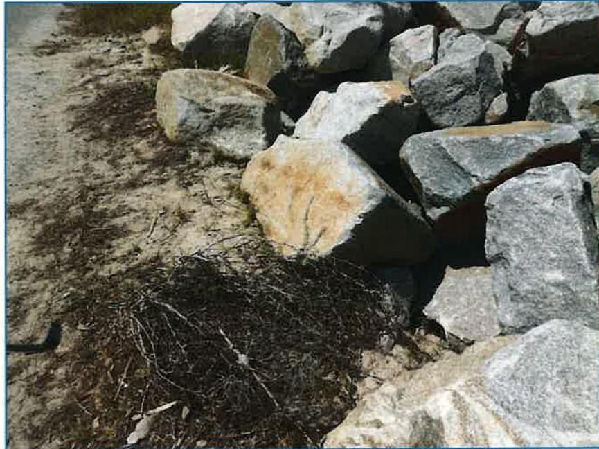
Photograph 5: Station 23+50 – Settlement of Stone Adjacent to Roadway
