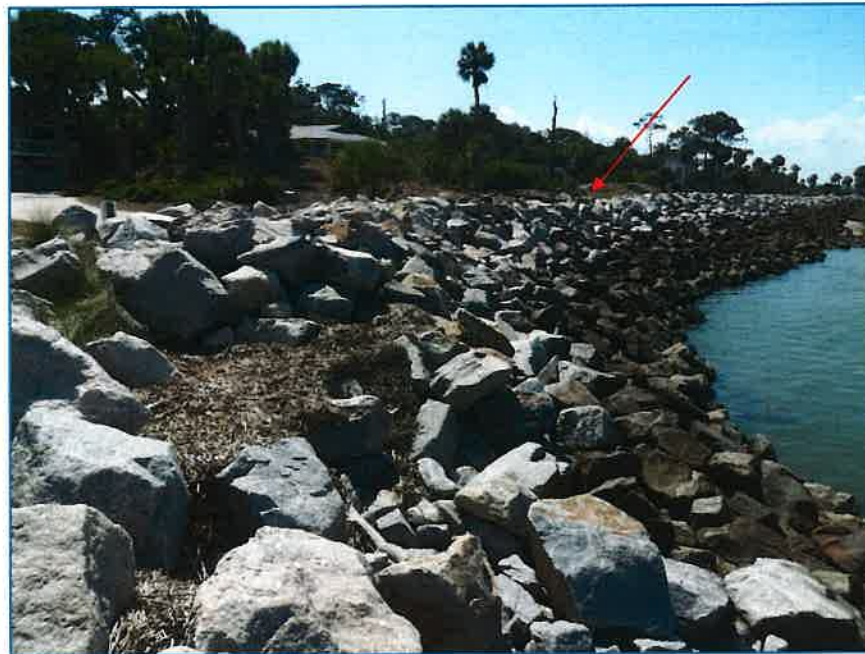
Photograph 6: Station 23+50 to 24+00 - Apparent Settlement of the Revetment
